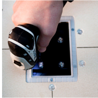
Remove the mud dam from the mounting platform
