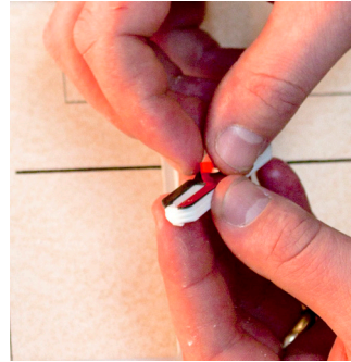
Peel red paper backing off base plaster shim and stack desired quantity on top of base shim
